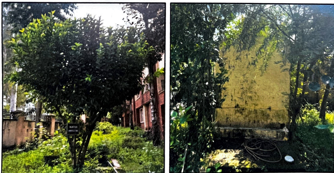
Figure 8: Rain Water Harvesting Tank
